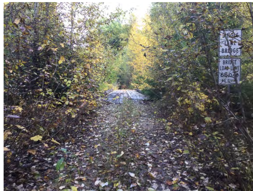
Approach from Left Bank when facing downstream
