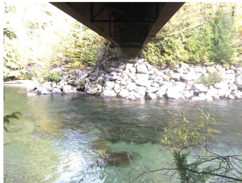
Right Bank Abutment when facing downstream
