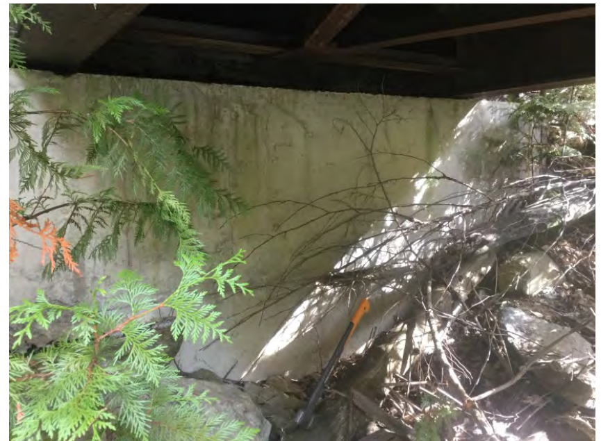
Right bank fill retainment structure
