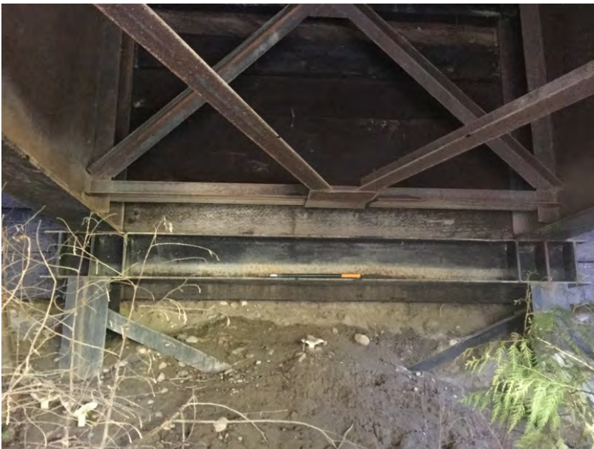
Left Bank Abutment when facing downstream
