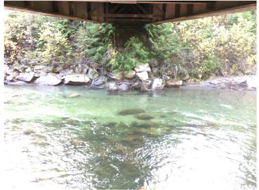
Left Bank Abutment when facing downstream
